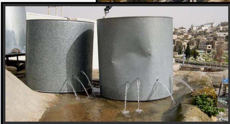
Left: A Palestinian families rooftop water tanks pictured after they were damaged in an attack by nearby Israeli settlers, Hebron. April 15th 2009.
